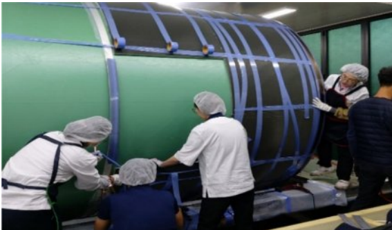
Fig. 13. Manufacturing of Sandwich Cylindrical Structure(2)
