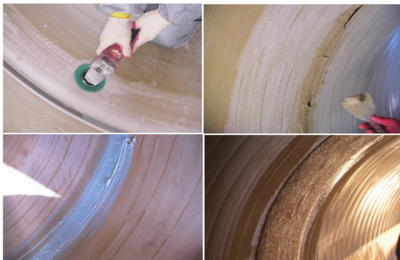
Fig. 16 Reinforcement by hand ray-up.
